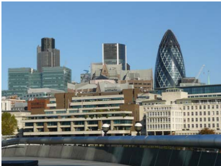
City of London (as seen from the DMAG office)
